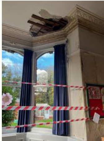
A/B - Signs of damp and damage to original plaster and joinery.
