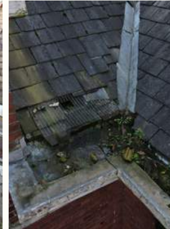
B - Insufficient drainage outlet and debris blockage.
