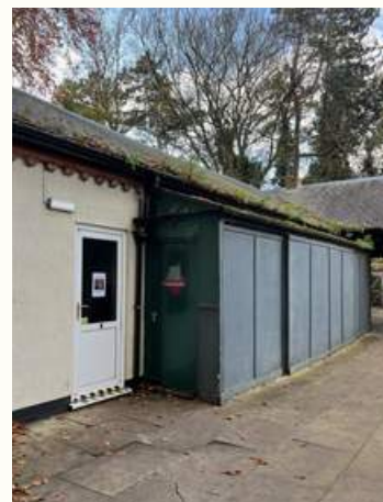
B: Modern lean to extension
