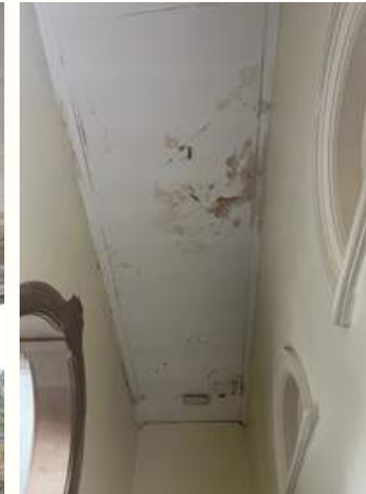
C/D - Evidence of internal cracking to ceiling/walls over lead roof.
