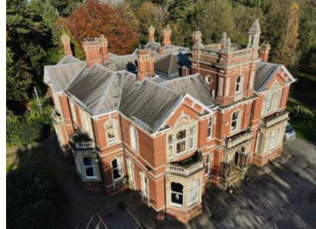
B - Main south elevation, view from above.
