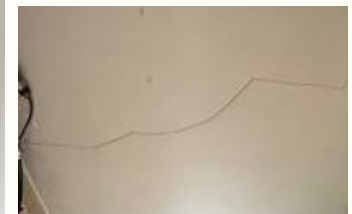
C/D - Evidence of internal cracking to ceiling/walls over lead roof.
