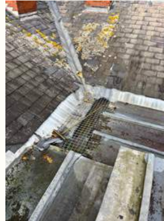
B - Insufficient drainage outlet and debris blockage.
