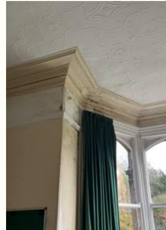
A/B - Signs of damp and damage to original plaster and joinery.
